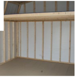
INSULATION SEEN FROM INSIDE THE STRUCTURE
